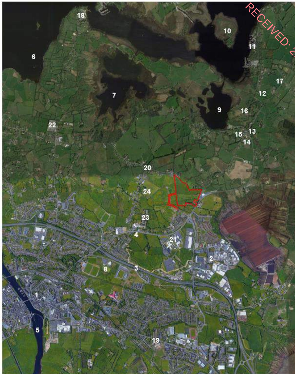
Figure 10-6: Aerial view with the site of the Proposed Development outlined in red in its broader landscape context. Viewing altitude: 11.00 km. Source: Google Earth
